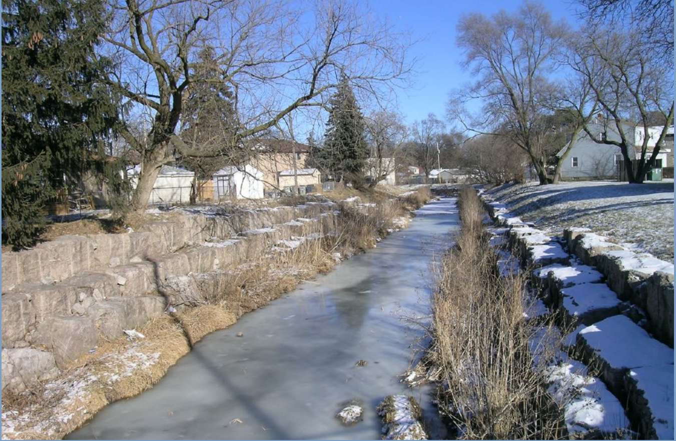
Today's neighborhood-Lincoln Creek near N. 60th St. & W. Custer Ave.
